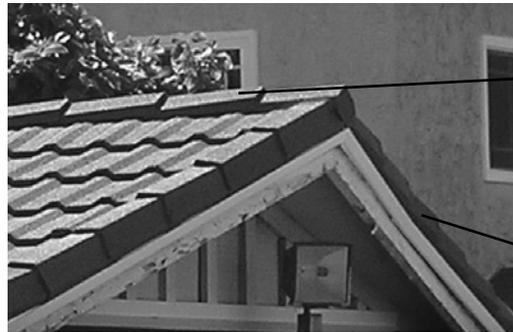
Two "C" channels stacked to form a 5" wide ridge beam.
