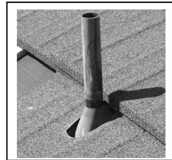
Tile section fitted over Flashing
