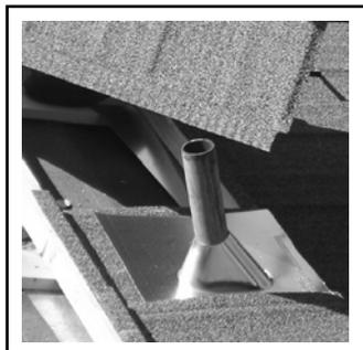
Full tile installed around pipe
